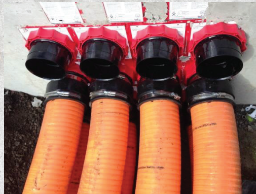
Connection of Hateflex flexible conduits using KES150-D system cover
