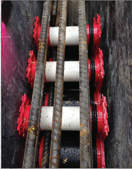
HSI150 & HSI90 wall inserts mounted in formwork
