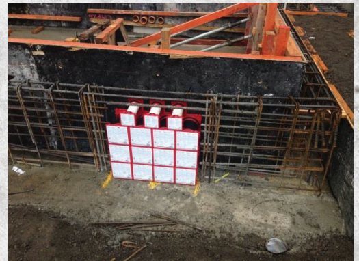
HSI150 & HSI90 wall inserts mounted in formwork
